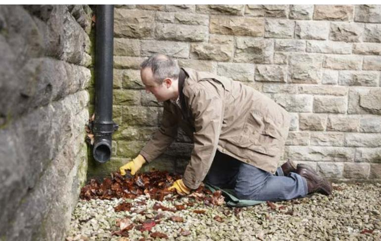
**Regular maintenance is the best way to keep a listed building in good repair. Keeping drains clear is a simple but effective way to prevent damp.**
