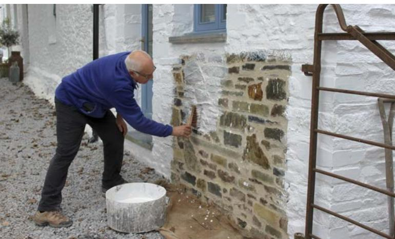
**It is important to use the appropriate materials in the maintenance and repair of listed buildings. Limewashing is a traditional and effective finish to protect buildings with solid walls.**
